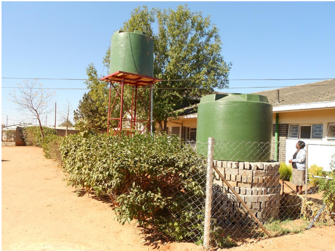
Above left is the recently installed tank
